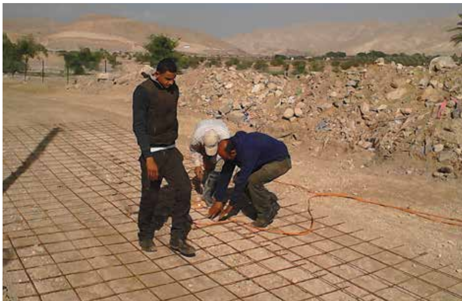
Strengthening of the road before concreting
