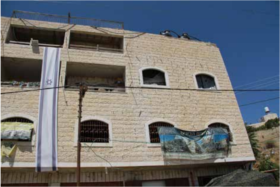
Al-Rajabi house, owned by the al-Rajabi family and occupied by Israeli colonizers and the Israeli forces in April 2014. (5 August 2016, BADIL)
